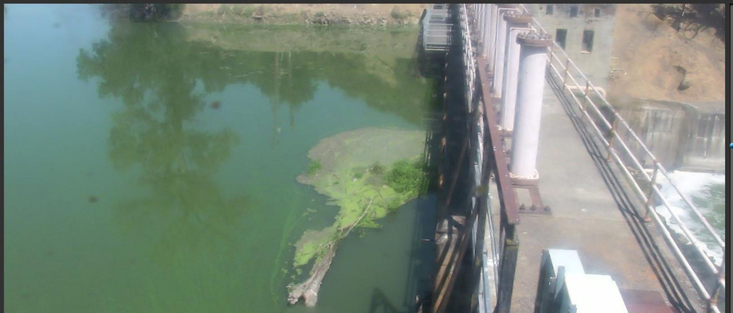
Cache Creek Dam: Source Water
