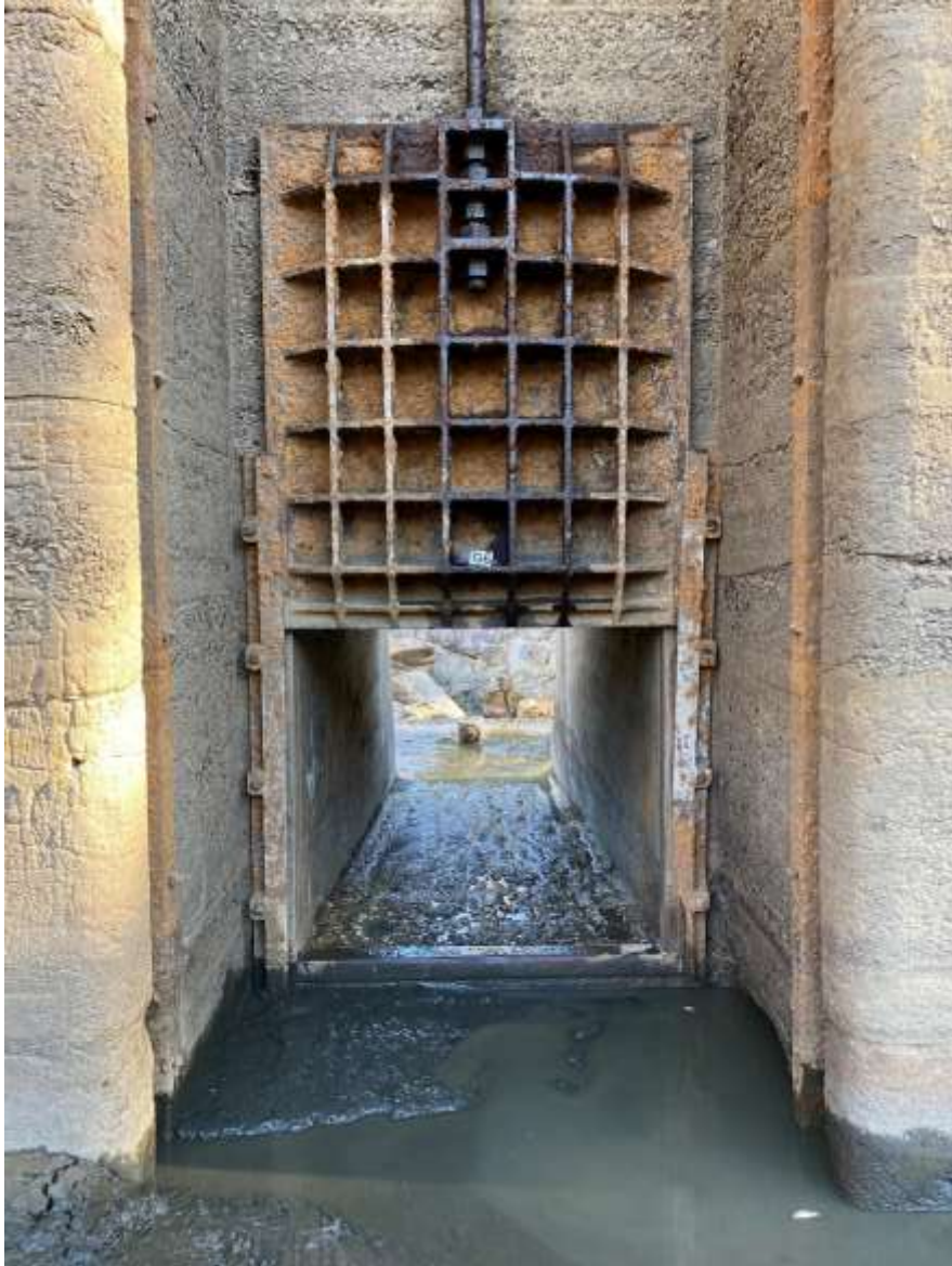
Cache Creek Dam – Gate 6
