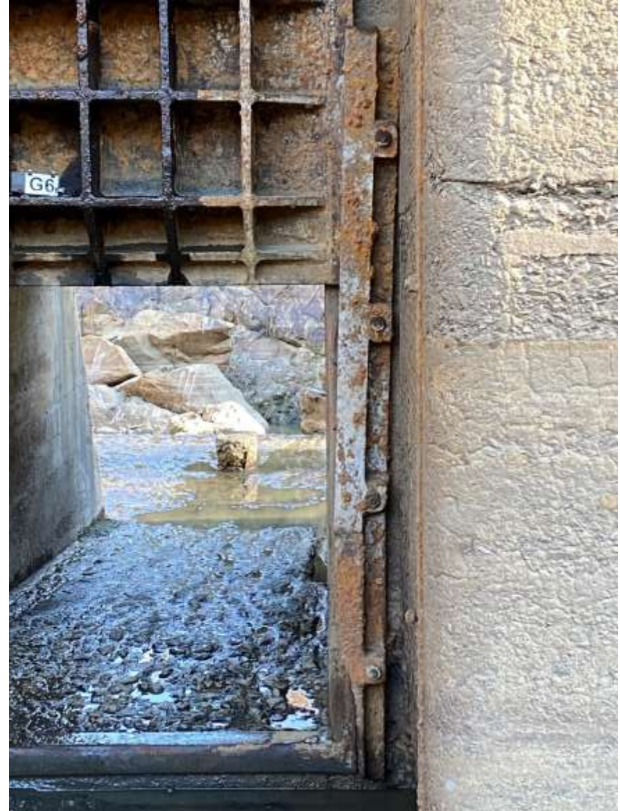
Cache Creek Dam – Gate 6 Right Z Bar
