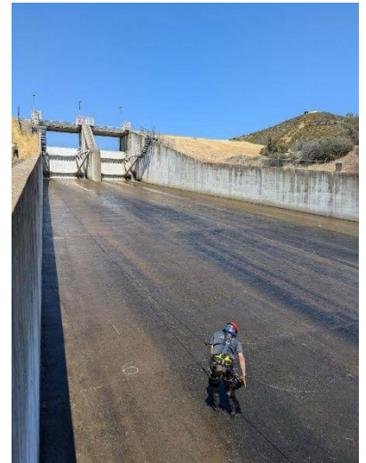
Photo of the IVR Spillway inspection on July 11, 2024.
