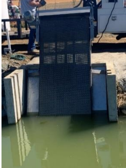
Photos of automated trash screen (middle) and mechanical removal of aquatic weeds (left and right).
